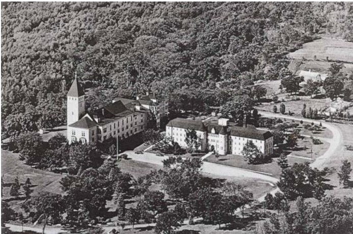
Villa Maria Academy South County Road #2 at Wells Creek
