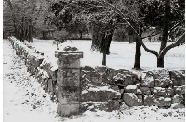
Winona Cottage Stone Wall Mortar Less Construction
