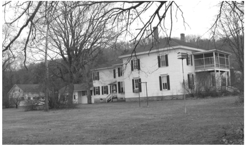
Dacotah Cottage Garrard Avenue between Dacotah and Burr Oak Streets
